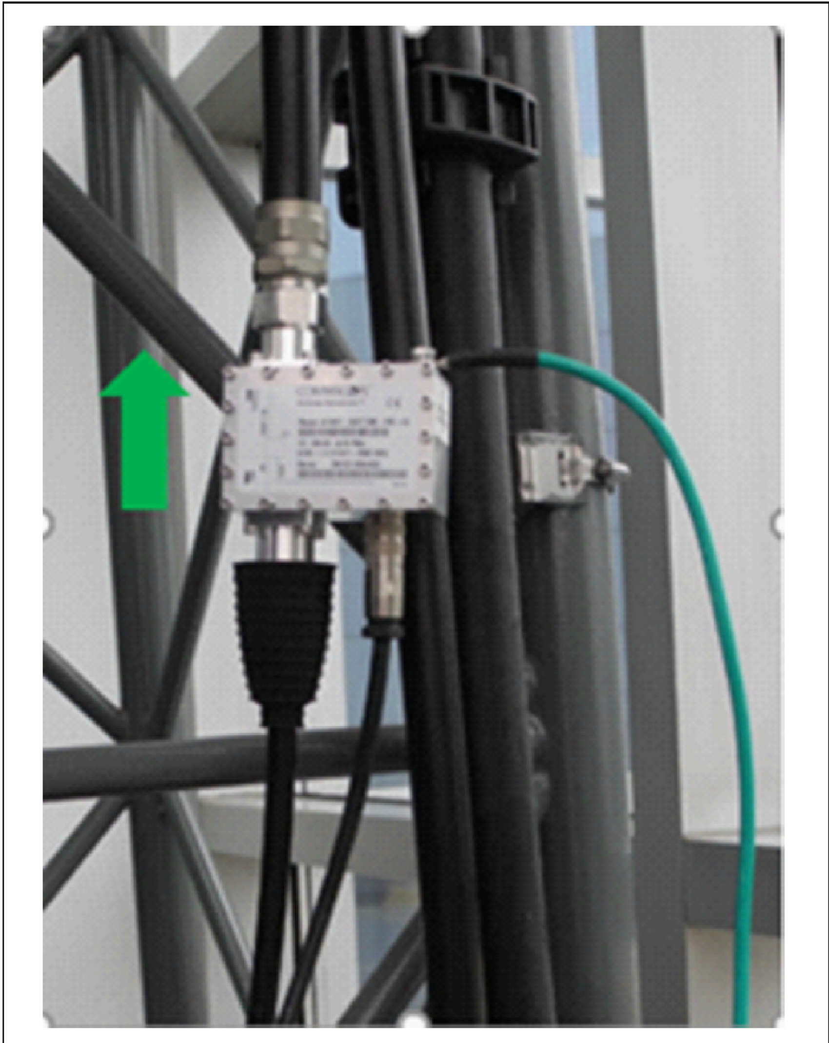
Figure 3. Recommended vertical position
