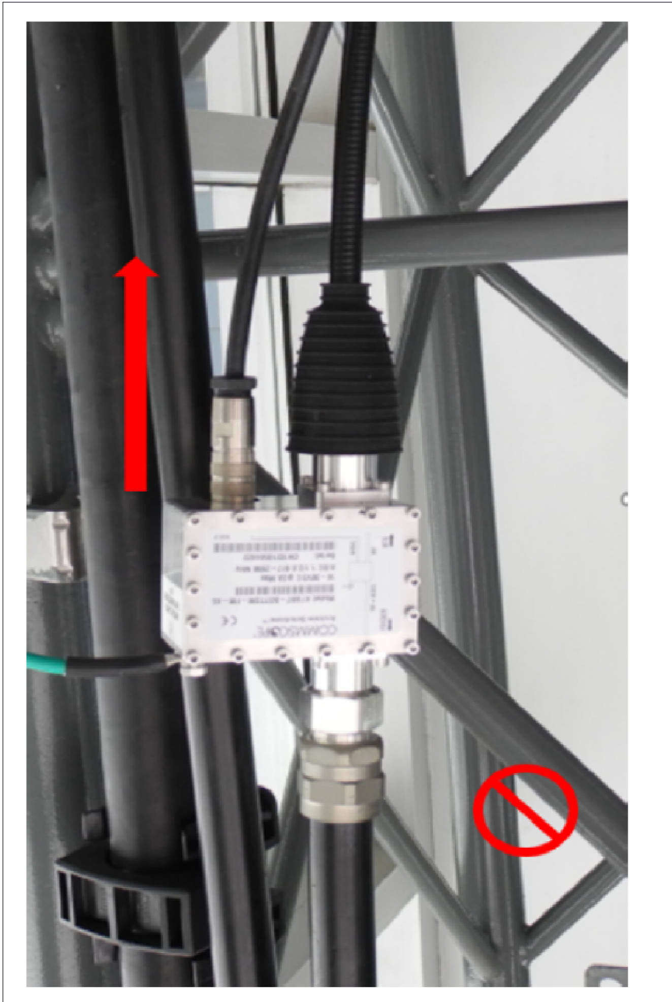
Figure 4. The AISG port facing up or tilt up is forbidden.
